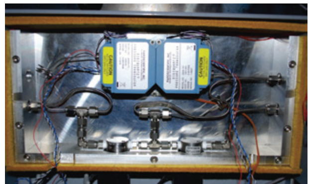
Figure 4. Pressure Sensors and Valves in Heated Enclosure.
