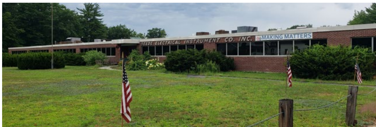
The remaining building of Beede Electrical Instrument Co. (now Faria Beede) in Penacook, NH.
